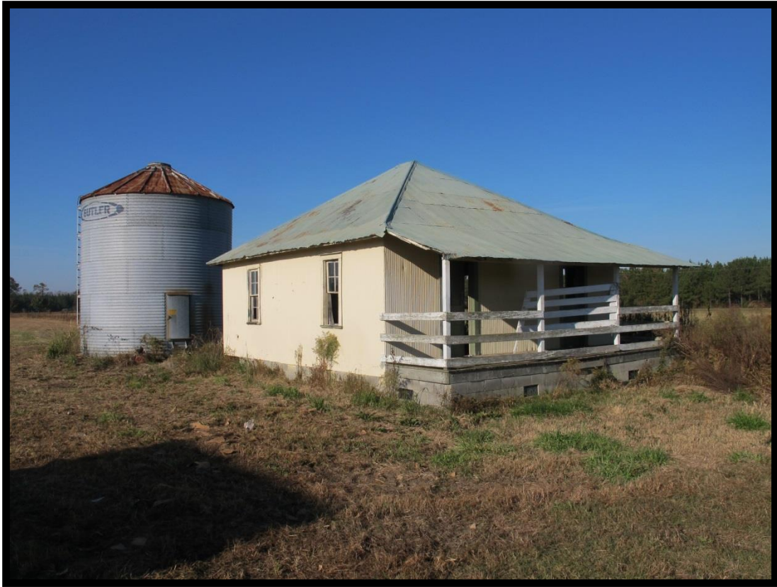
Figure 18: (Former) Byrd Store Office (# 017), Looking Northwest.
