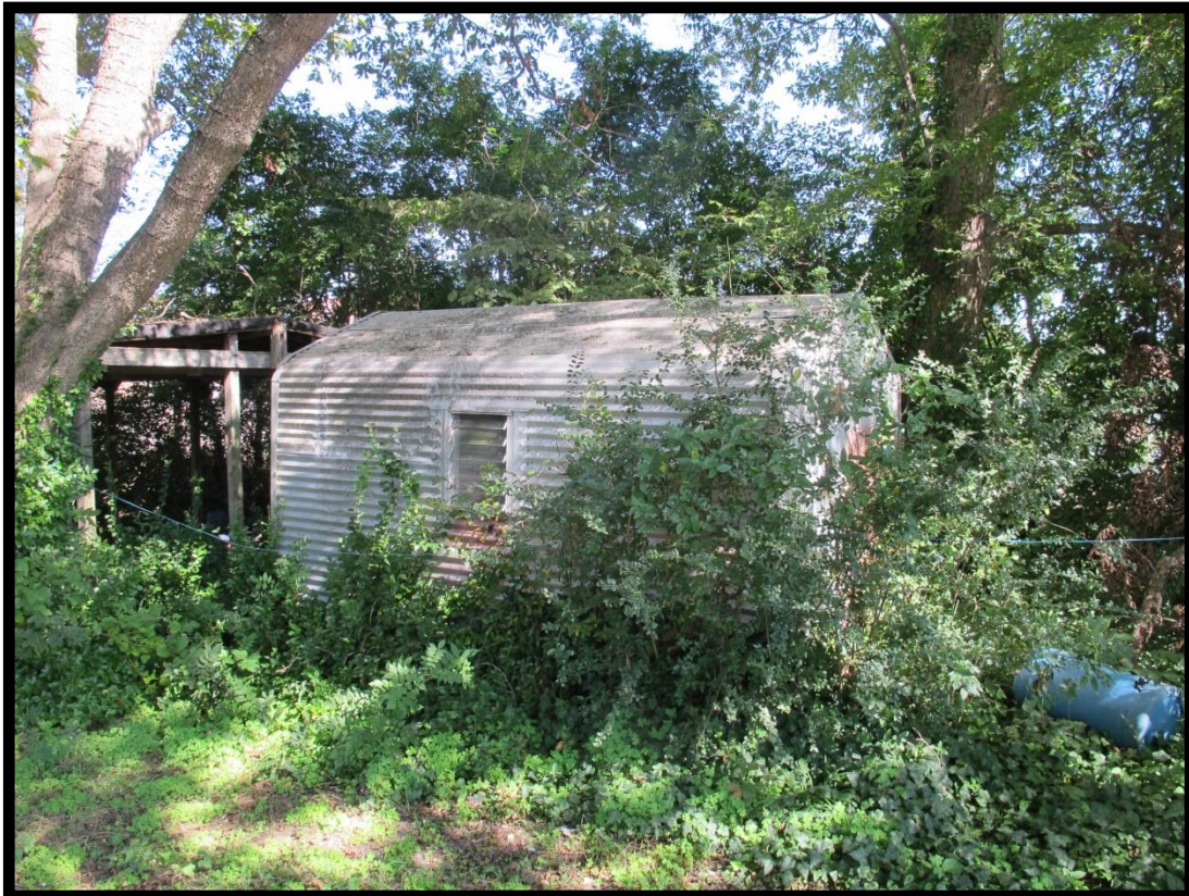
Figure 58: James A. Smart House (# 025), Garden Shed Looking Northeast.
