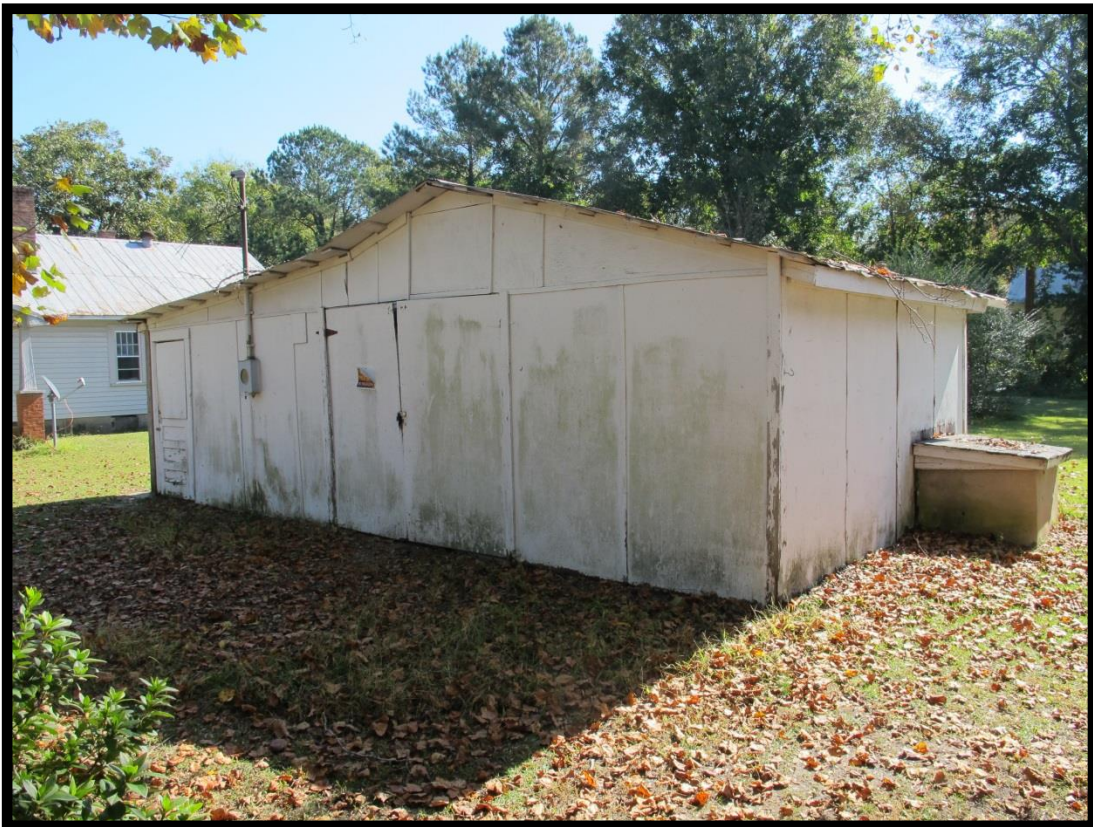
Figure 33: House (# 021), Outbuilding/Garage Looking Southeast.
