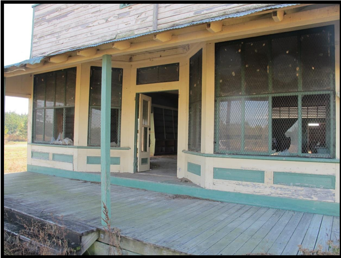
Figure 16: (Former) Byrd Store (# 017), Detail of Storefront Looking South.
