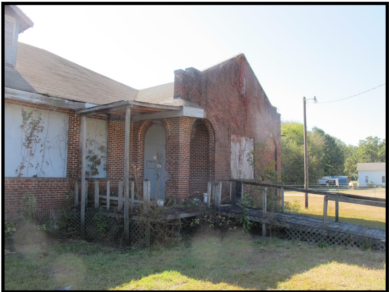
Figure 61: (Former) Bunnlevel Elementary School (# 026), Detail of Entrance Looking Southwest.
