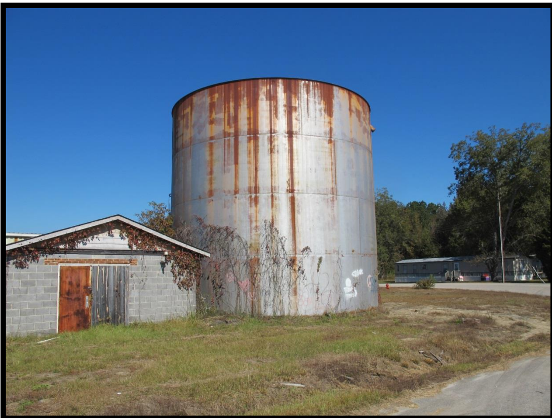
Figure 67: (Former) Bunnlevel Elementary School (# 026), Storage Tank Looking Northeast.
