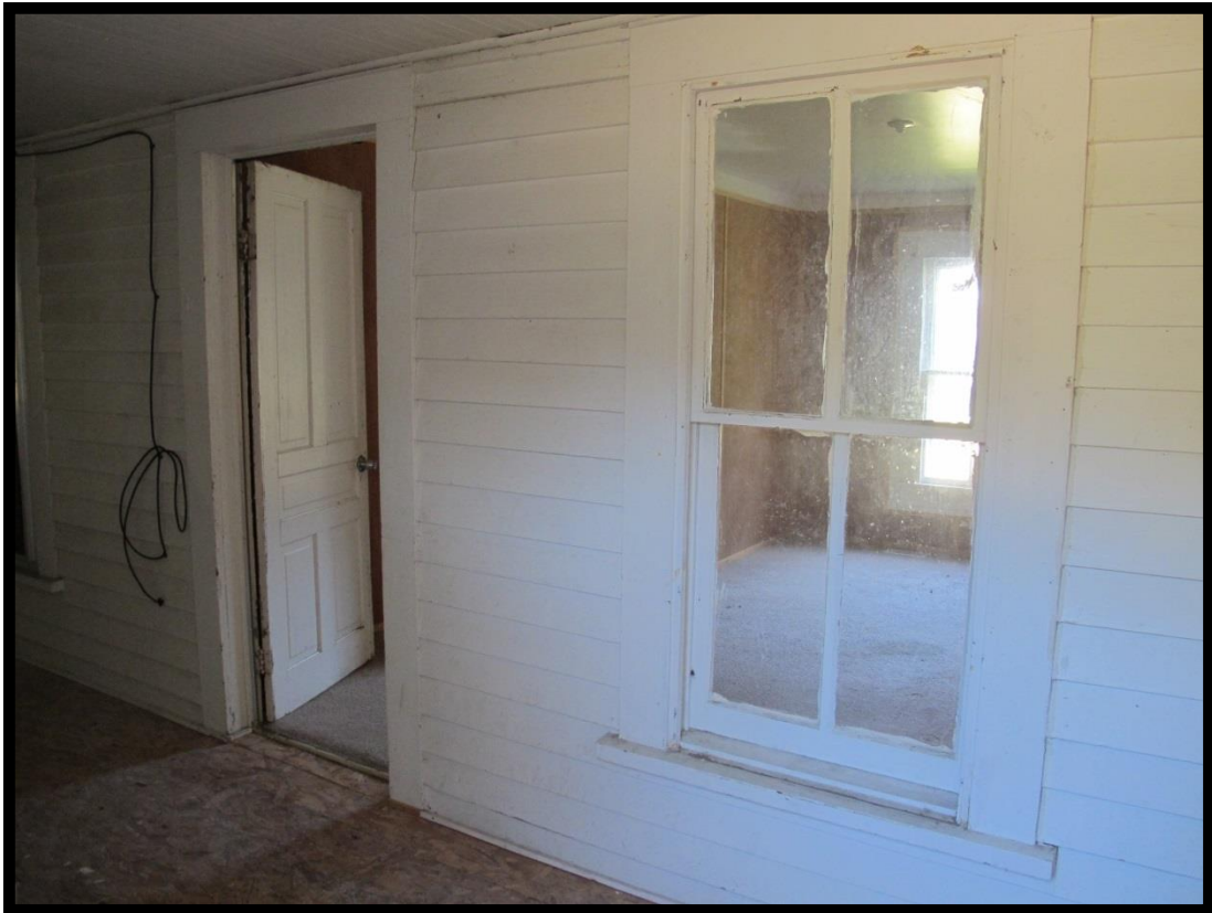
Figure 32: House (# 021), View of Enclosed Porch.
