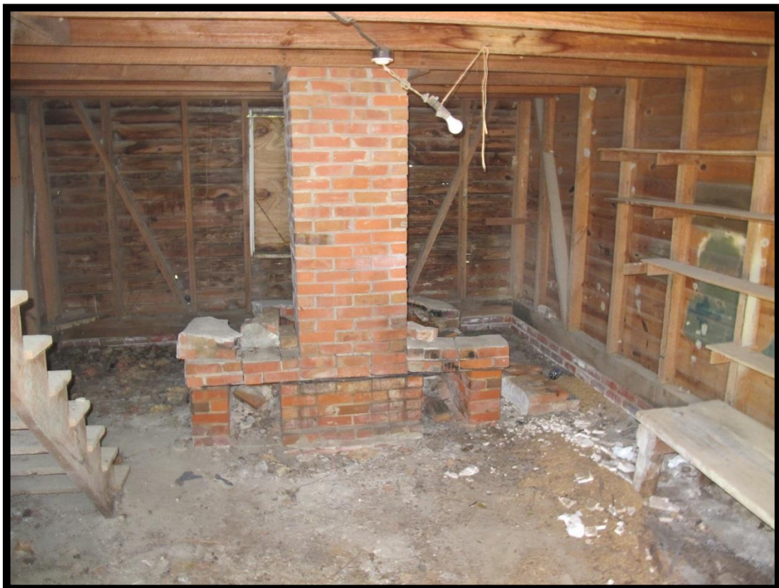
Figure 43: House (# 022), Interior of Central Section of Outbuilding Looking East.
