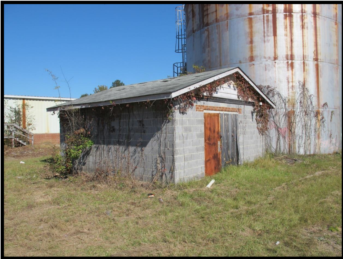
Figure 66: (Former) Bunnlevel Elementary School (# 026), Outbuilding Looking Northeast.
