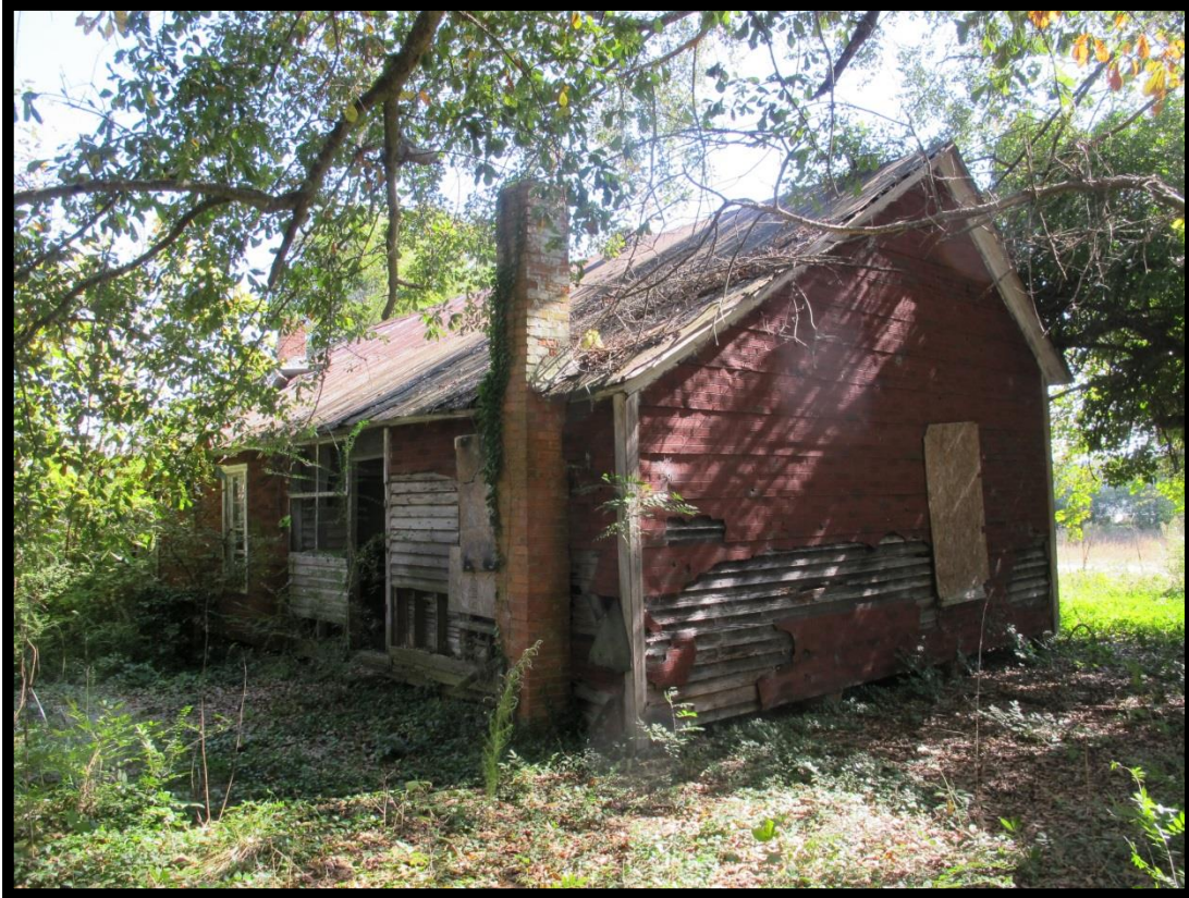
Figure 51: House (# 024), Looking Southeast.
