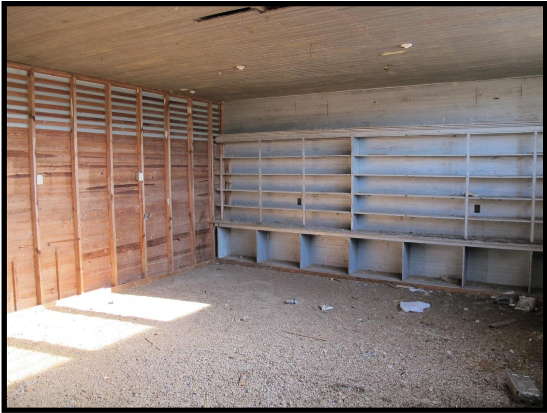
Figure 20: (Former) Byrd Store (# 017), Interior of Storage Room Looking North.
