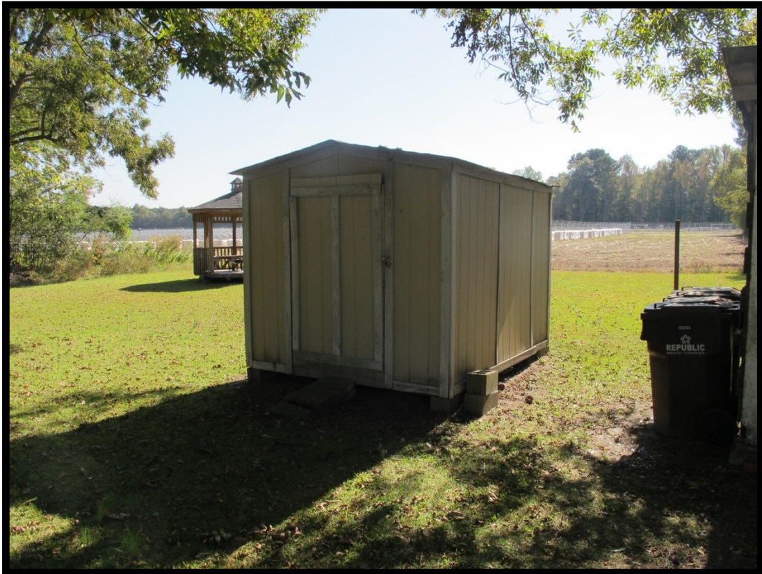
Figure 48: Stella S. Williams House (# 023), Outbuilding Looking Southeast.
