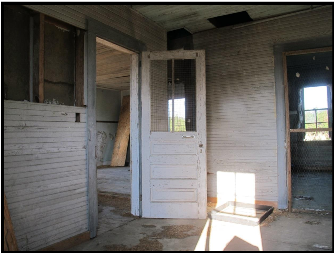
Figure 21: (Former) Byrd Store Office (# 017), Interior Looking Northwest.
