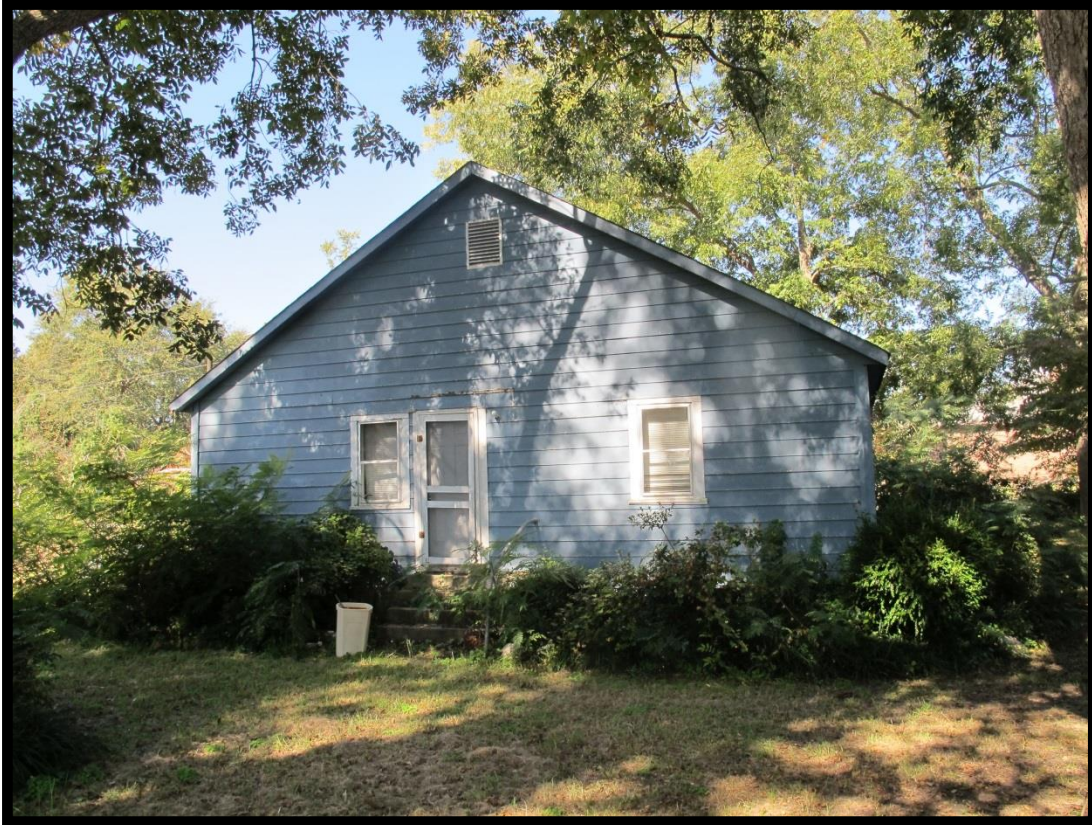
Figure 57: James A. Smart House (# 025), Looking Northwest.
