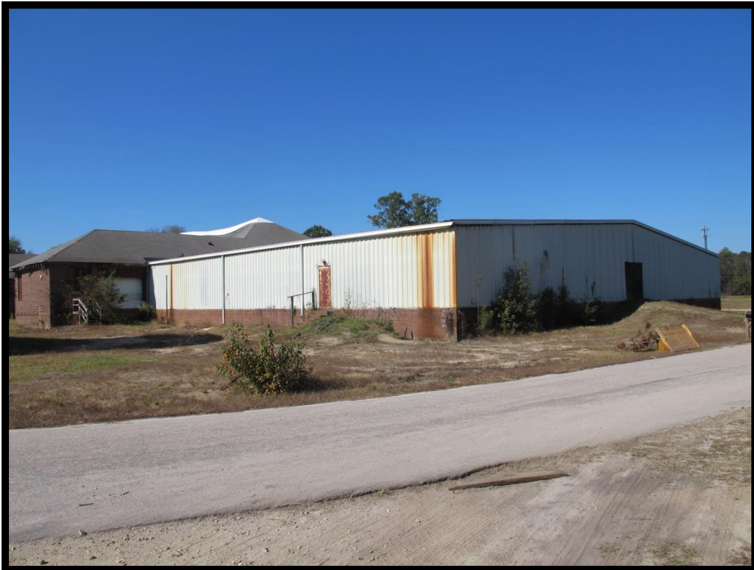
Figure 65: (Former) Bunnlevel Elementary School (# 026), Addition Looking Northwest.
