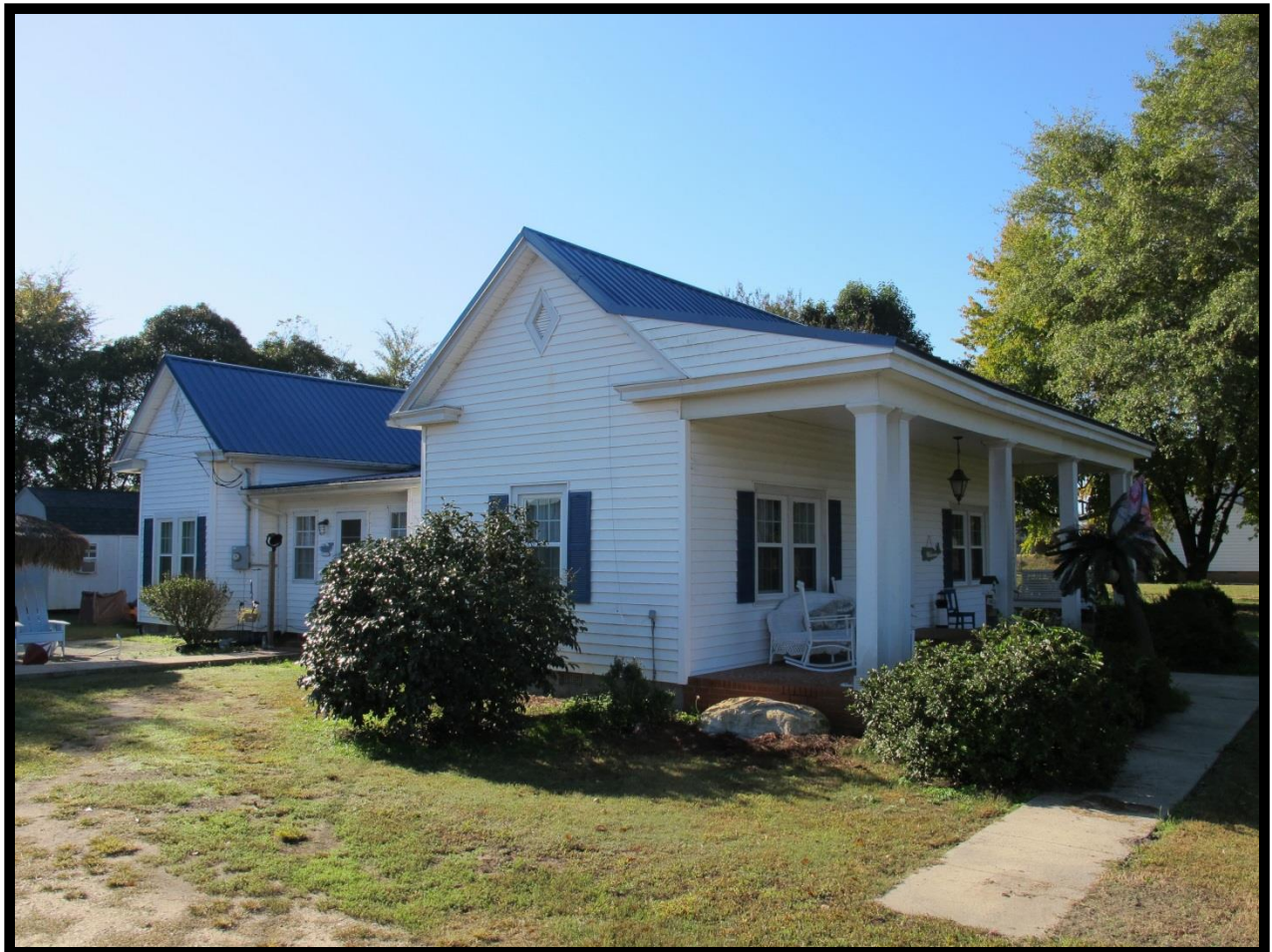
Figure 5: Lemuel D. Byrd Jr. House (# 006), Looking South.
