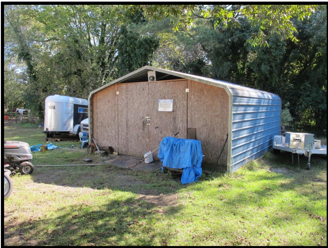
Figure 71: House (# 027), Enclosed Carport Looking Southeast.
