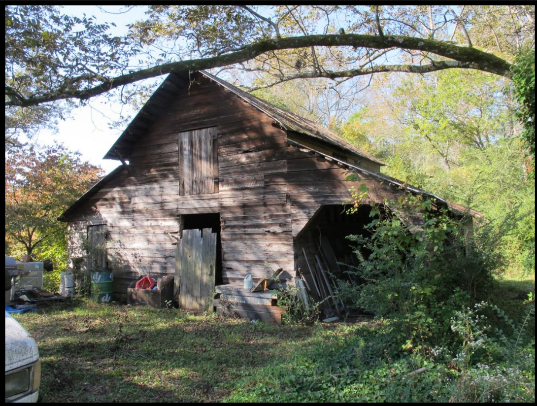
Figure 85: Frank D. Byrd House (# 041), Outbuilding Looking Southwest.
