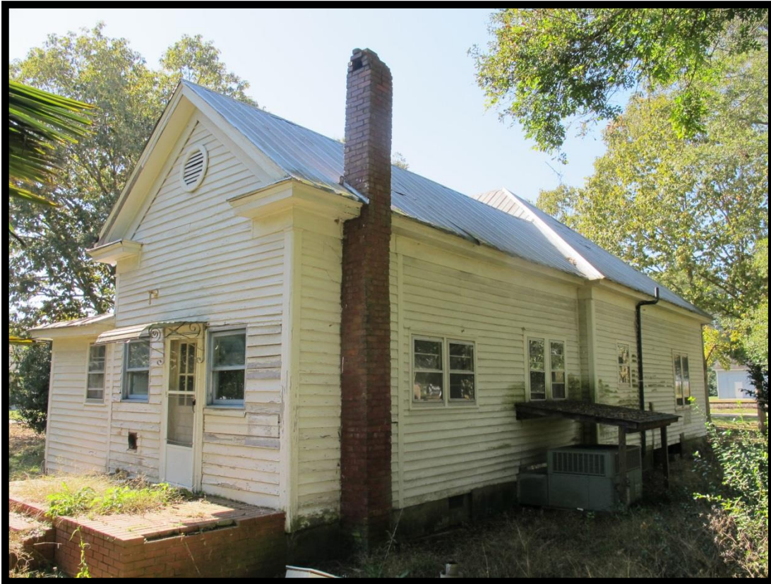
Figure 36: House (# 022), Looking Southwest.
