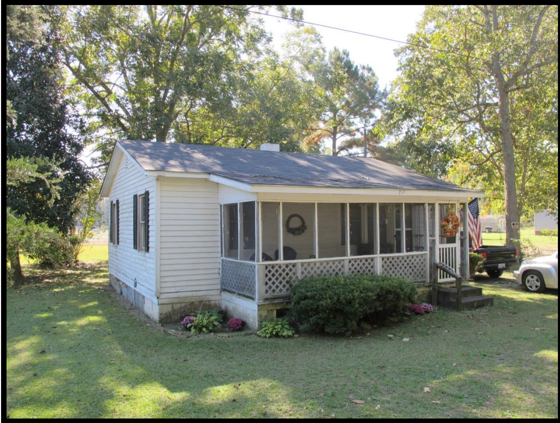
Figure 45: Stella S. Williams House (# 023), Looking South.
