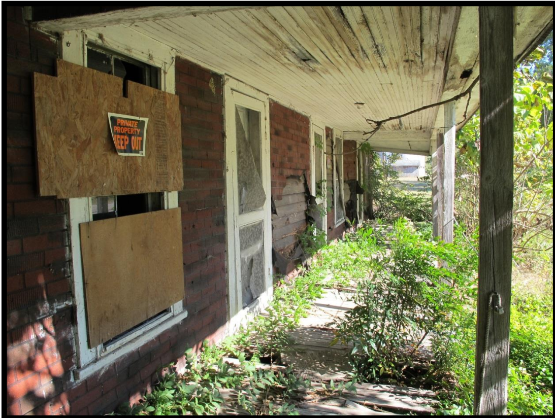
Figure 52: House (# 024), Detail of Southeast (Front) Elevation Looking Northeast.
