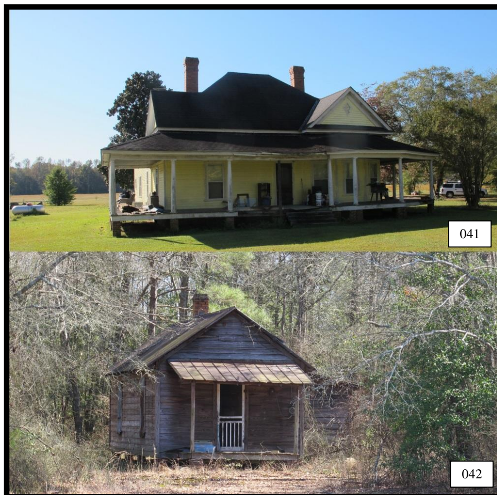
Figure 80: Frank D. Byrd House (# 041), Looking Southwest, and Byrd Tenant House (#042), Looking East.
