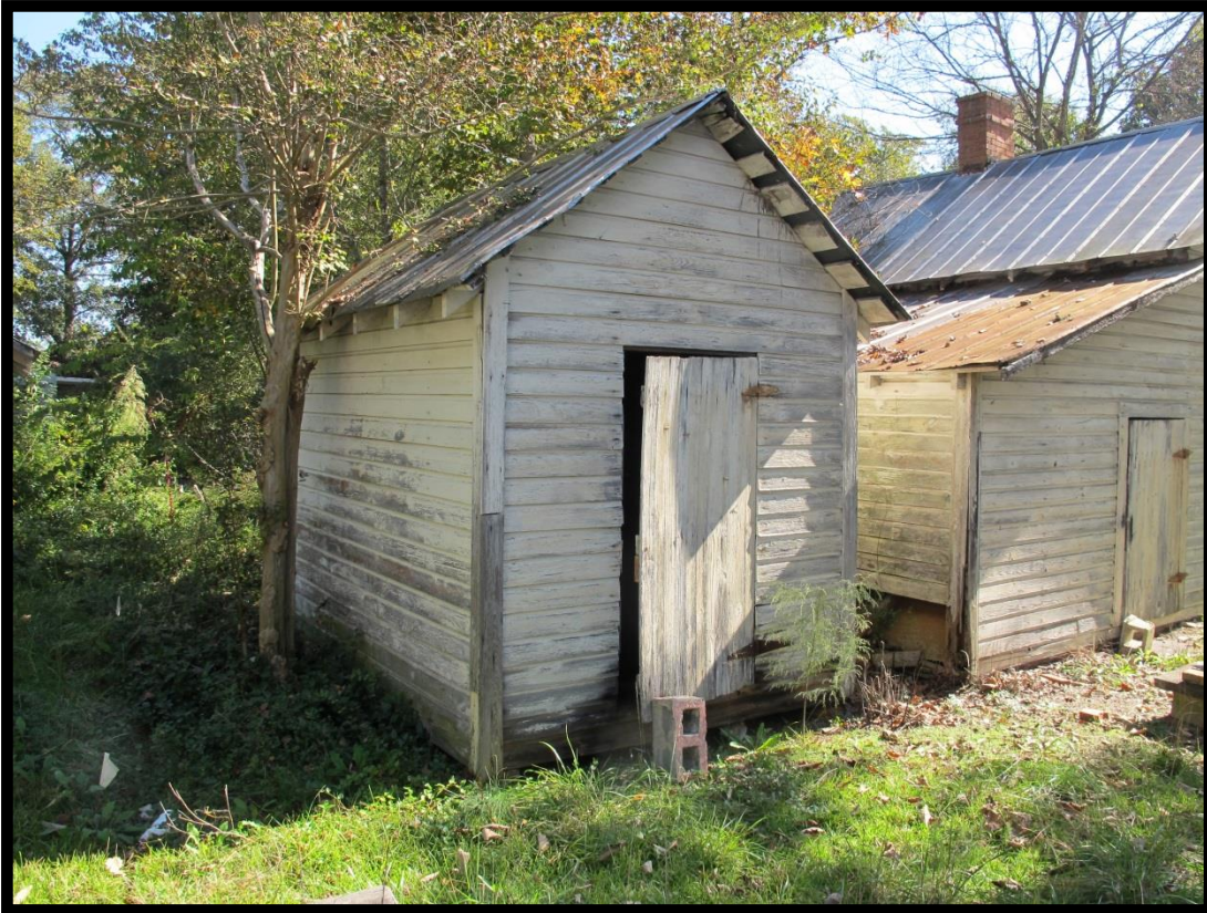
Figure 40: House (# 022), View of Frame Shed Looking East.
