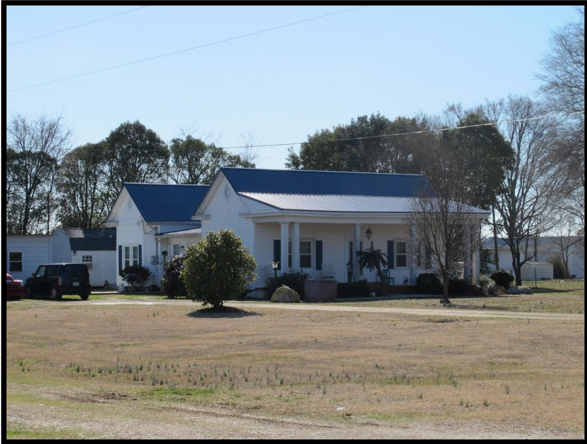
Figure 3: Lemuel D. Byrd Jr. House (# 006), Looking South.
