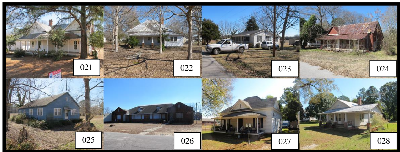
Figure 24: Resources in the Bunnlevel Historic District.
