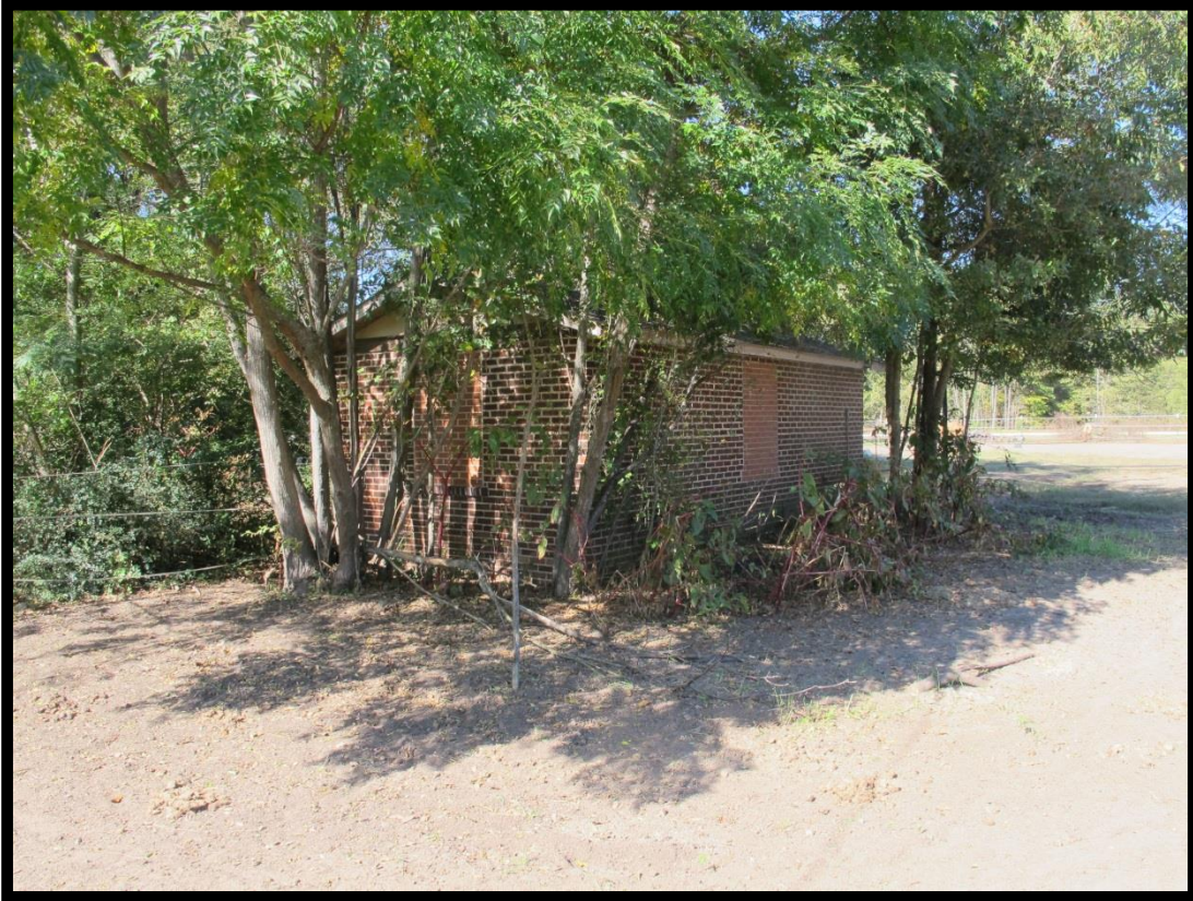
Figure 64: (Former) Bunnlevel Elementary School (# 026), Pump House Looking Northwest.
