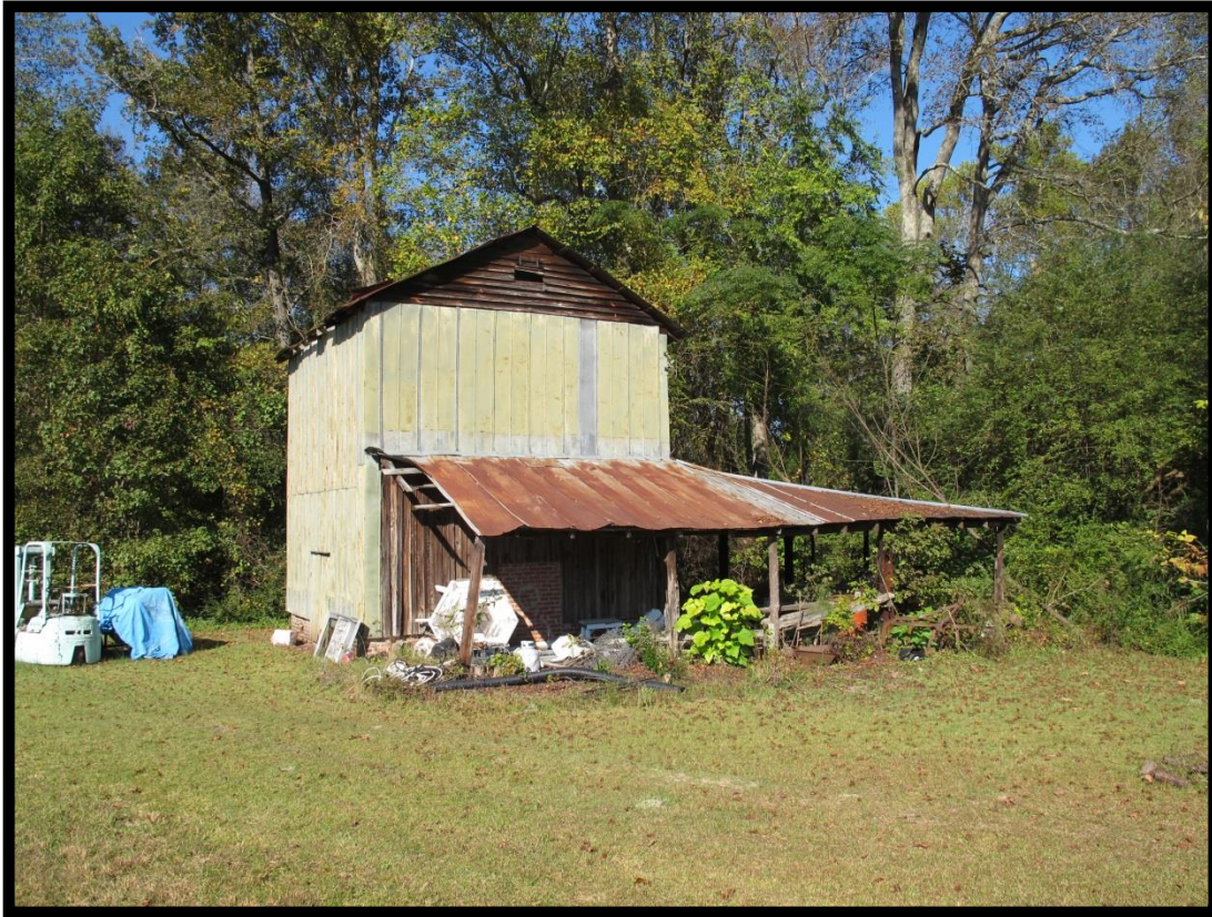
Figure 86: Frank D. Byrd House (# 041), Tobacco Barn Looking Northwest.
