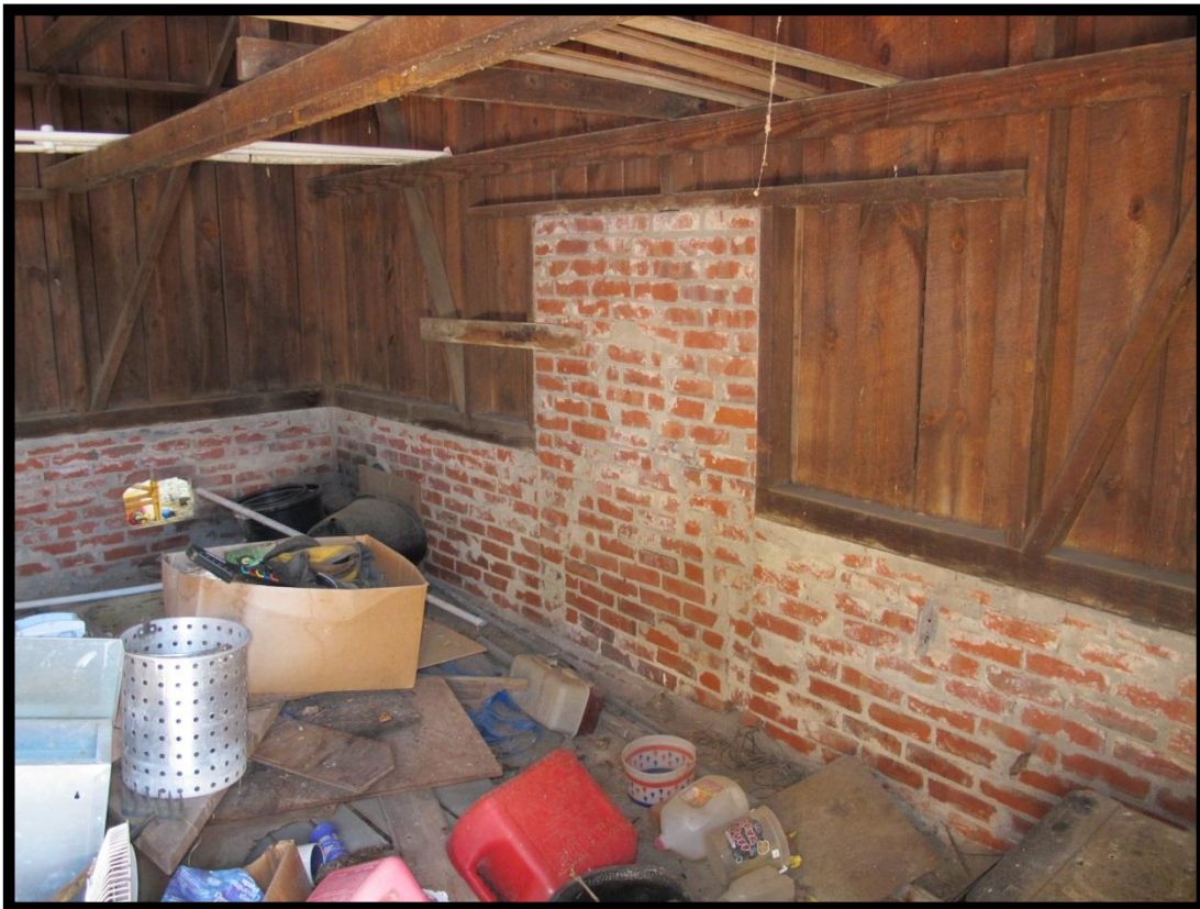
Figure 87: Frank D. Byrd House (# 041), Interior Tobacco Barn Looking Northeast.
